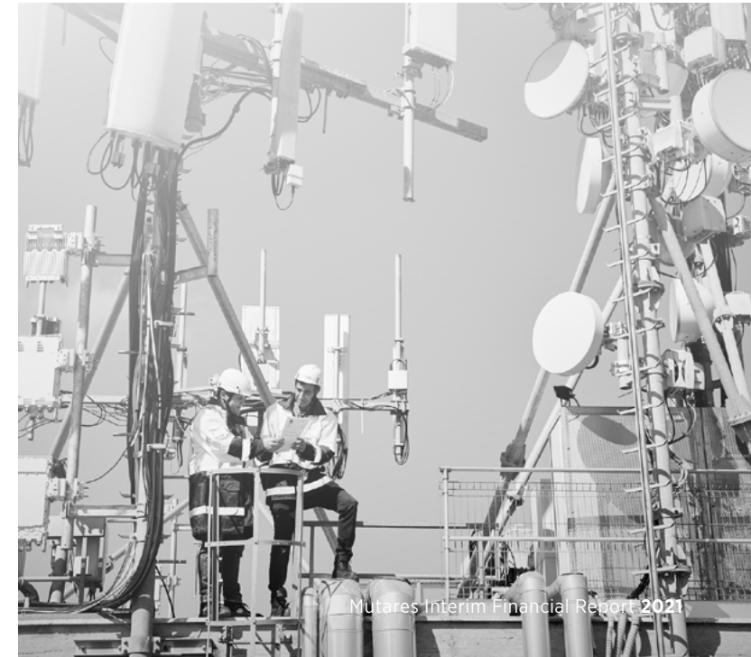
Employees during maintenance on site
