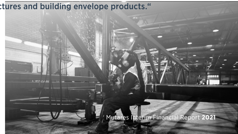
Manufacturing parts for a highway bridge
